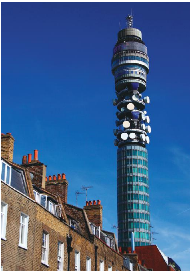
Telecommunications tower in London
